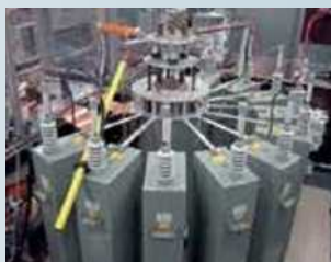
Surge current generator for generation of test impulses
